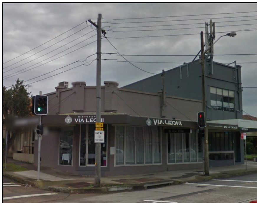
Photo 5: The corner property to the north west of the subject site.
